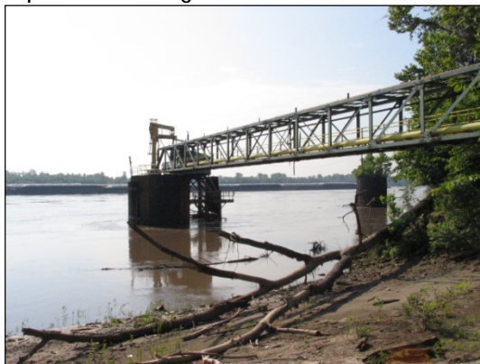
Liquid Bulk Mooring
